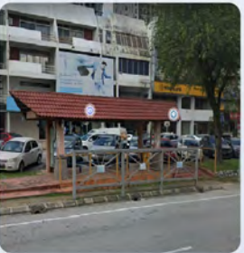
Bus stop at SS15 Maybank / RHB
