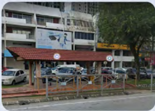
Bus Stop at SS15 Maybank / RHB
