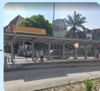
SS15 LRT STATION (GATE B BUS STOP)
