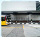
TAYLOR'S LAKESIDE CAMPUS (BLOCK B)
